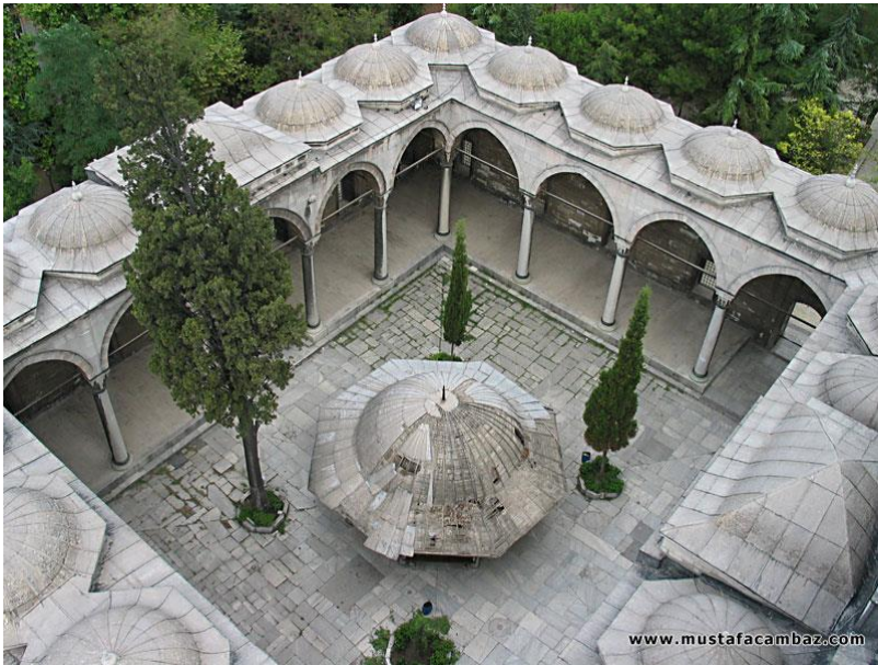
Figure 2. The yard containing a water tank with fountain 31
