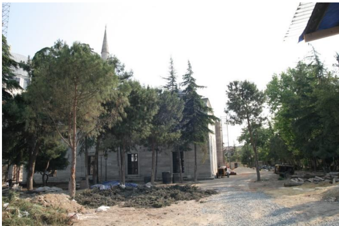
Figure 4. A view of the Islamic social complex landscaping restoration work
