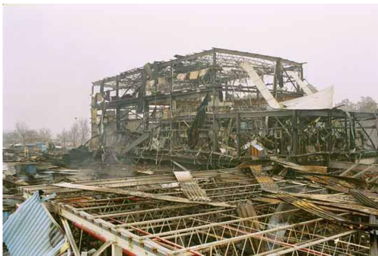
Figure 6: Dust explosion in North Carolina-WEST industrial plant
