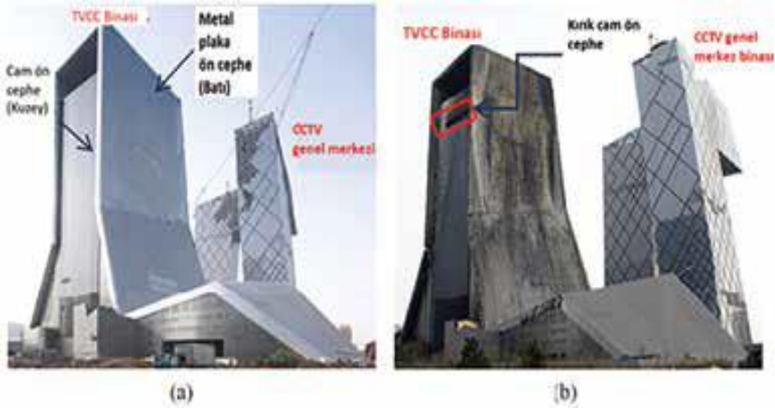
Figure 3. (a) TVCC building before fire, (b) TVCC building after fire
