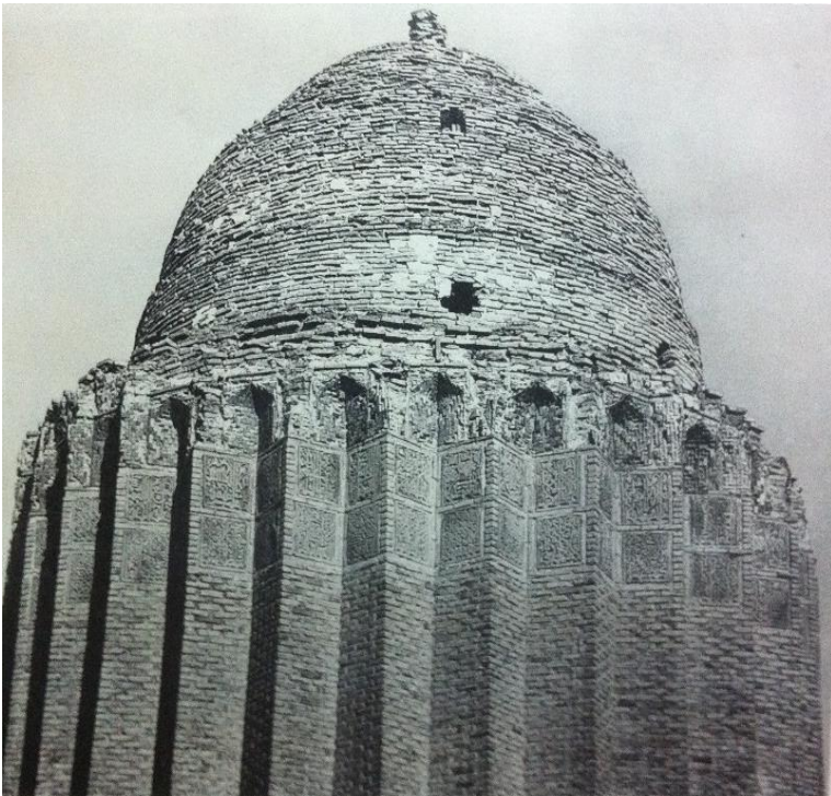
Figure 11. The dome cornice of the tomb (Wilber, 1955)
